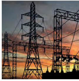
CRITICAL POWER SUPPLY
